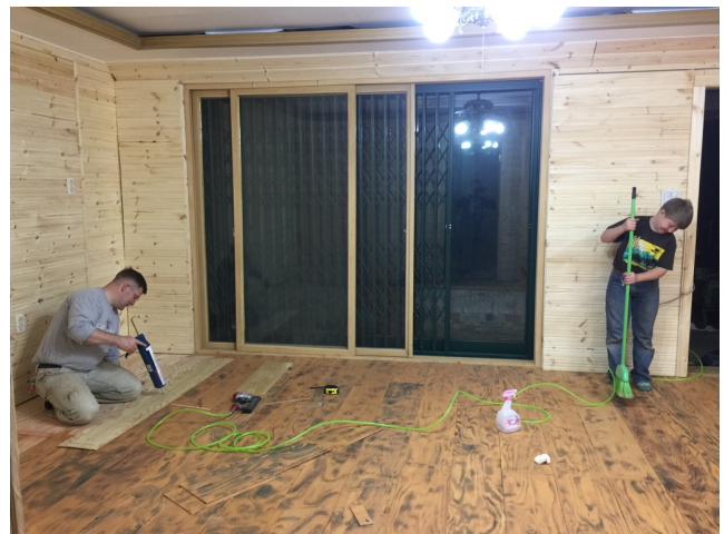
Remodeled a fellow missionaries house with handmade wood flooring.
